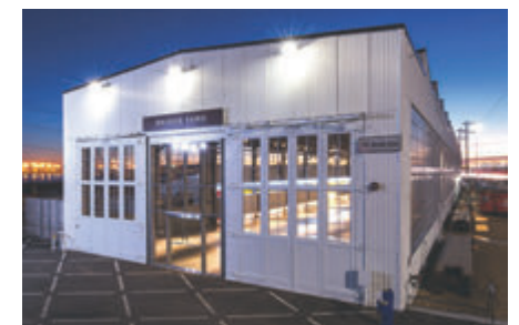
The Bridge Yard Building Former maintenance facility for the Key System electric passenger trains.
